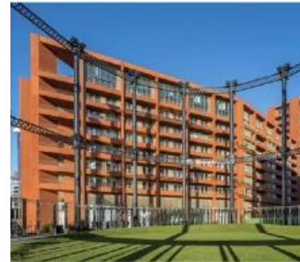
Kings Cross Central – design & engineering across 15 sites
